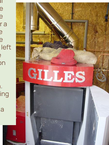
From field to boiler. Willow harvested, dried and chipped to feed into a woodchip boiler that heats the farmhouse.
